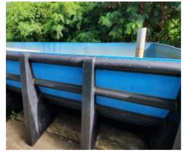
10 Ton Reservoir Tank
